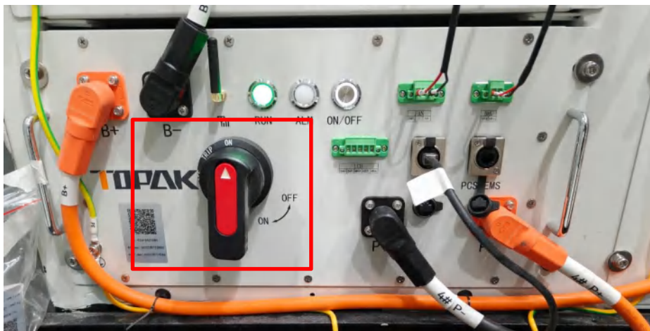
Diagram of switch in high voltage box
