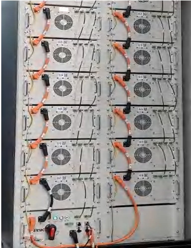
Schematic diagram of communication and power cable between PACKs
